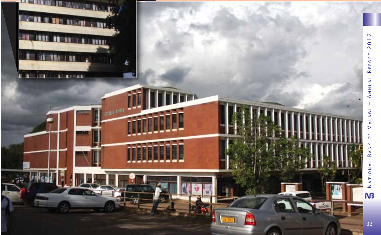
MPICO office complex City Centre, Lilongwe.
