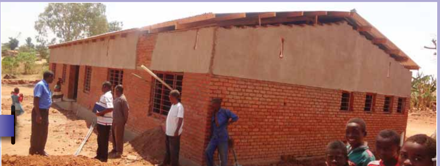
Construction of a MK10 million Maternal Clinic underway in Ntcheu
