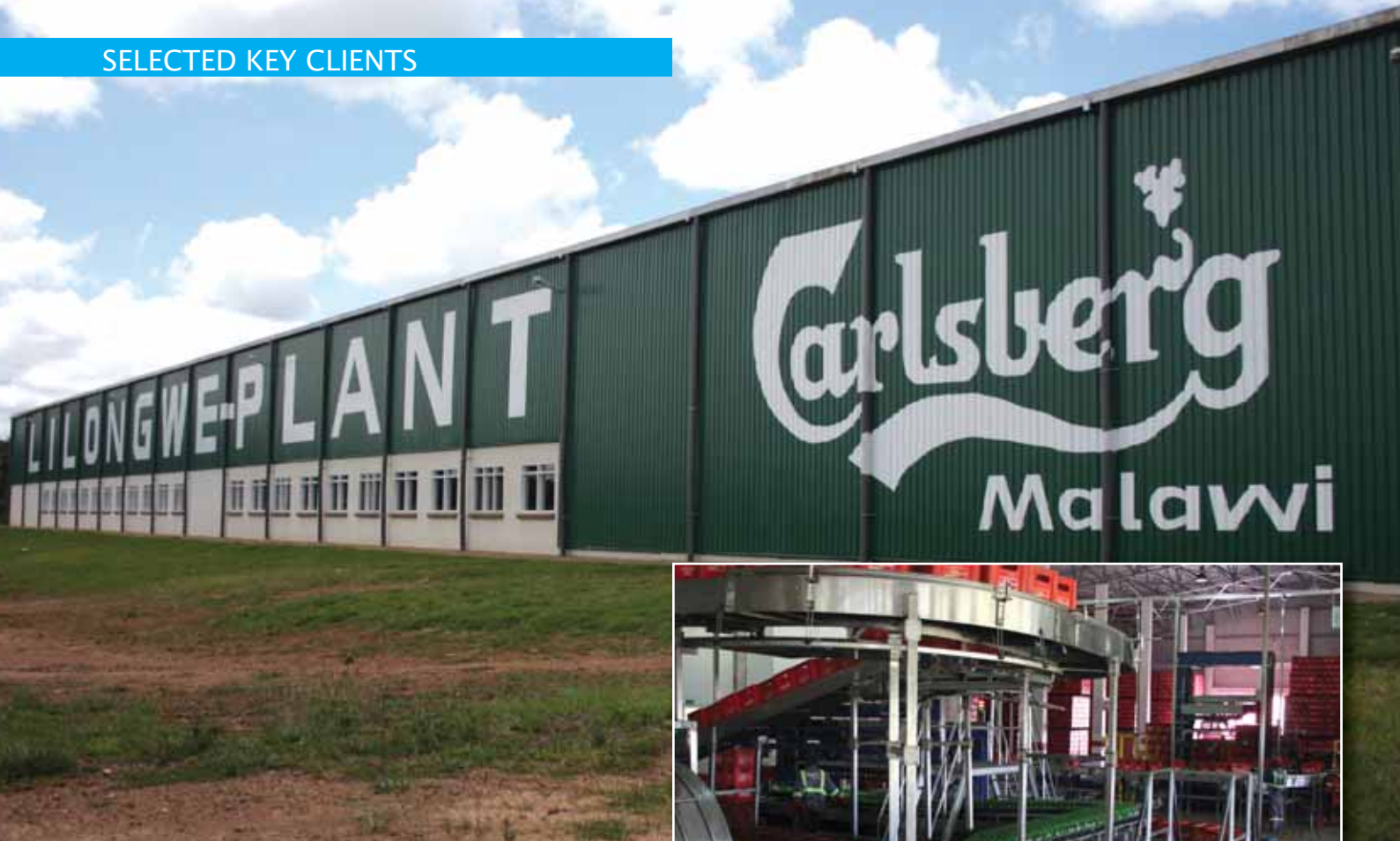
BBGL, Lilongwe new plant
