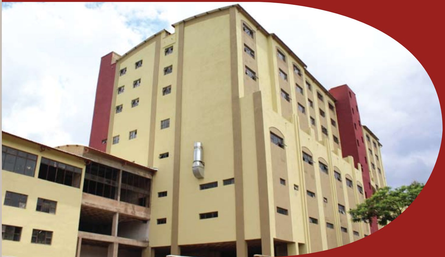
Crossroads Hotel under construction in Blantyre
